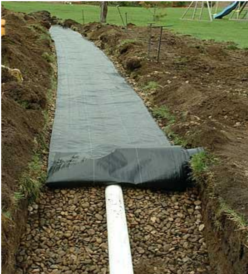
Figure 3-15: Example Infiltration Trench (source: North Dakota State University)
