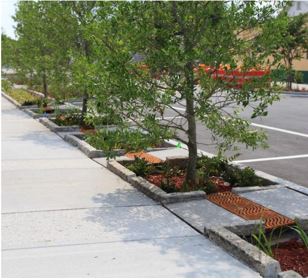
Figure 3-17: Surface visual of a Boulevard Tree Cell installation (source: City of Portland)
