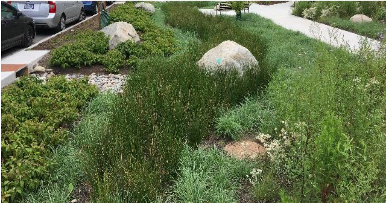
Figure 3-18: Example Bioretention Unit (Source: City of Vancouver)
