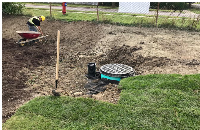
Figure 12. Rain garden catchbasin outlet
