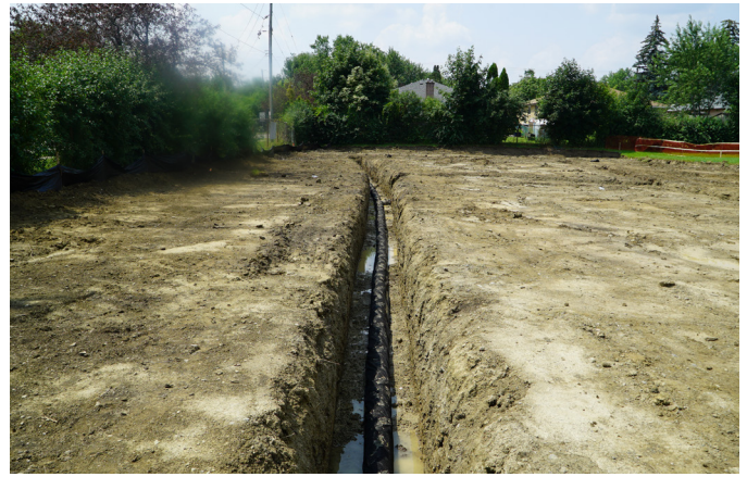
Figure 8. Vegetation removed, underdrain trench excavated
