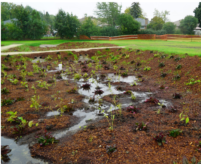
Figure 15. Ponding water over the surface of the first cell of the rain garden
