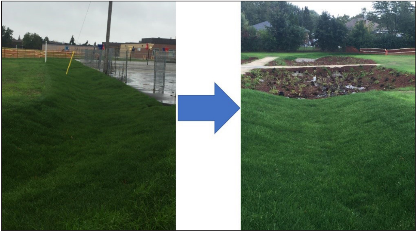
Figure 14. Conveyance of sheet flow via grass swale to the cell of the rain garden
