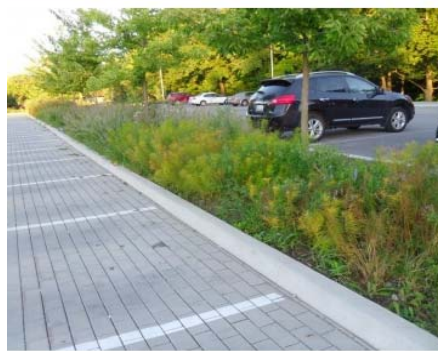
parking lot bioretention sharing underground reservoir with adjacent permeable paving, Edwards gardens, Toronto
