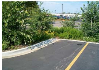
The sunken curb holds the edge of the asphalt pavement and lets water freely flow to the bioretention cell beside the 7sigma parking lot in Minneapolis, MN (USA)
