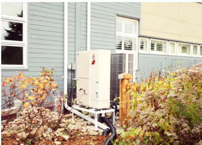
Figure 1. The outdoor fan coil for the Mitsubishi Zuba ASHP used in this study.
