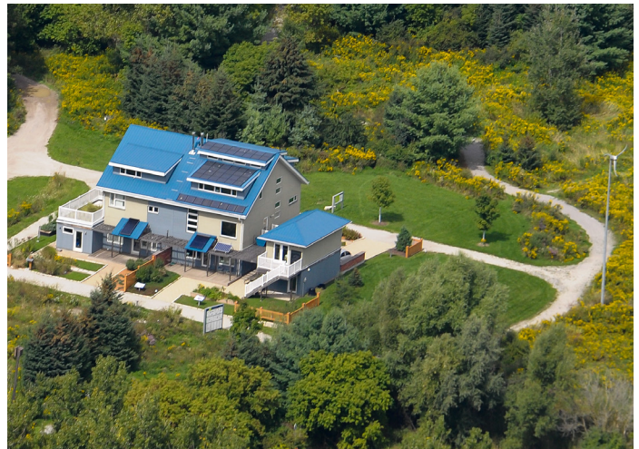
Figure 2. The Archetype Sustainable House A (left) and House B (right) with roof-mounted solar PV and adjacent wind turbine.
