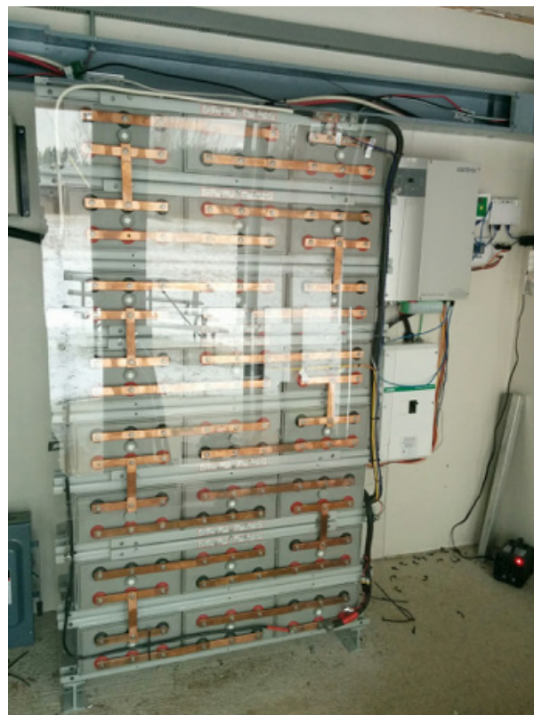
Figure 3. The 1600 Ah lead acid battery bank with its protective plastic shielding is shown on the left. The Xantrex XW inverter and Combox are mounted to the right of the battery bank.
